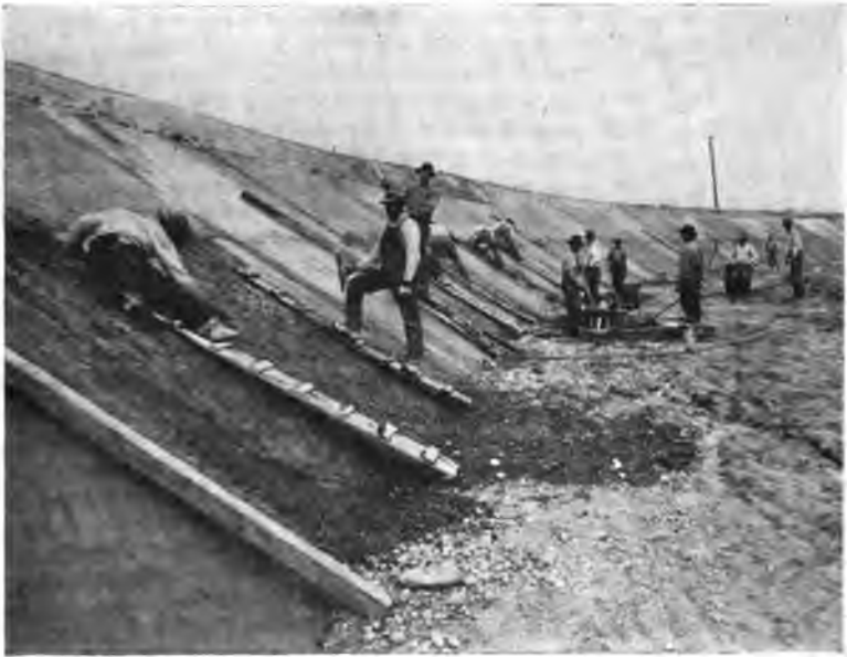
FIG. 84.—Lining Canal with Concrete, Idaho.
